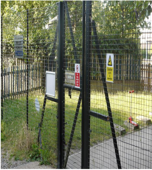
Rear pedestrian gate
